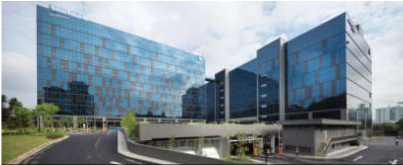
Completion of a 11-storey Hi-Tech Building (Phase One) and a 8-storey Hi-Tech Building (Phase Two)
