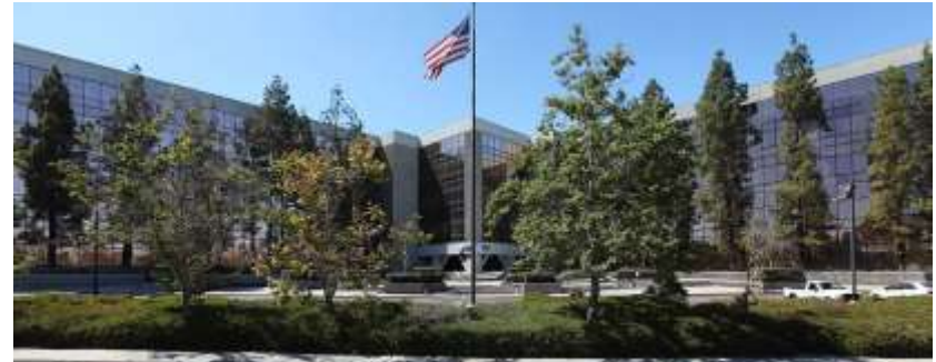
40:60 joint venture with the Sponsor to acquire 14 data centres in US
